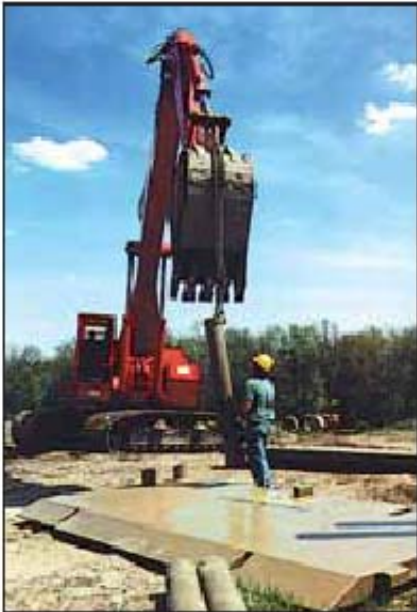
Excavator positioning trench shield components for job site assembly.
