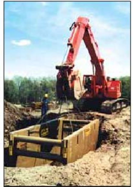
The fully assembled trench shield is lowered into position.
