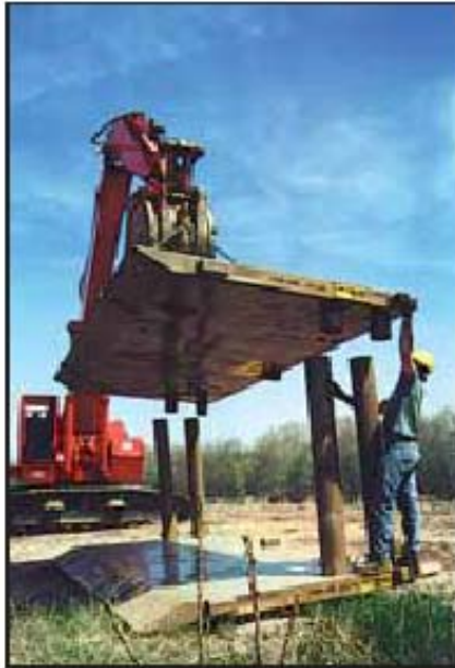
Final assembly of shield components is completed at ground level.
