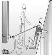
8) What is this lanyard called? \_\_\_\_SELF-RETRACTING\_\_\_\_\_\_
